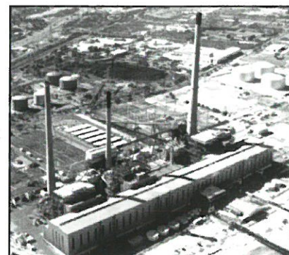
Kwinana power station, or, more correctly, energy station. This station has used oil, coal and natural gas as fuel in its lifetime.
